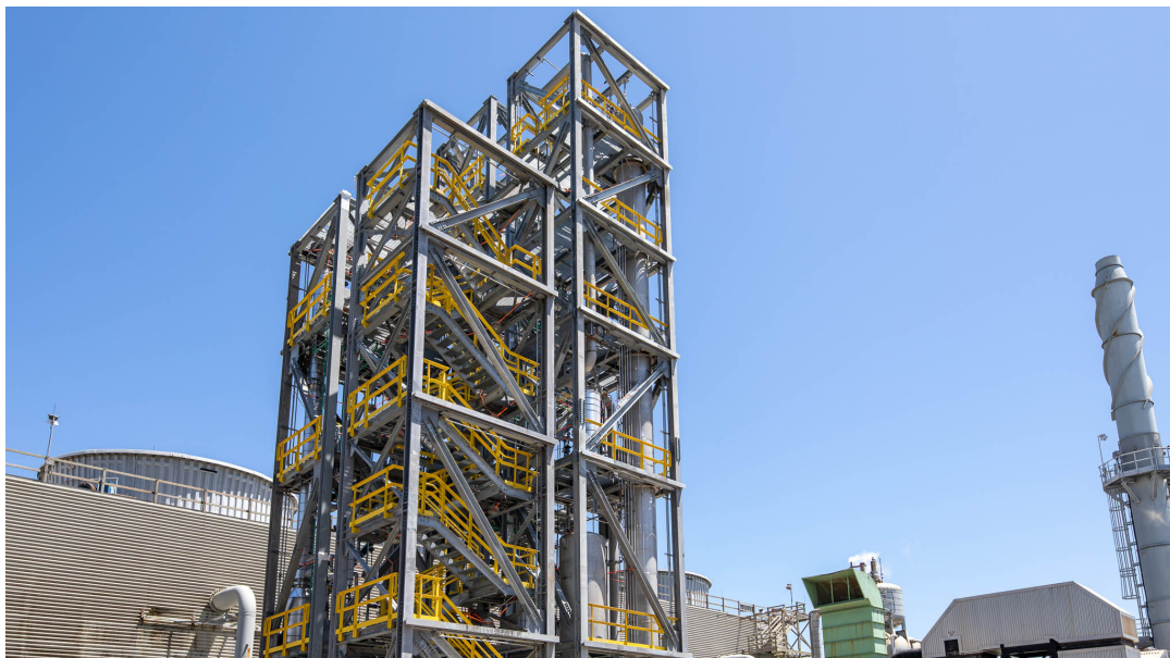
Los Medanos Energy Center | Pittsburg, California
